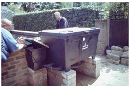
12. Pumps in place and working.
