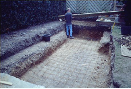
1. Excavations complete with wire reinforcements
