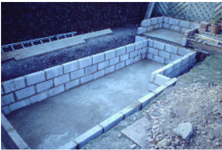
5. Breeze blocks in place leaving room to back-fill with cement
