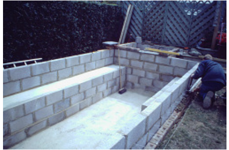
8. Bricklaying the outer wall (note wire ties)
