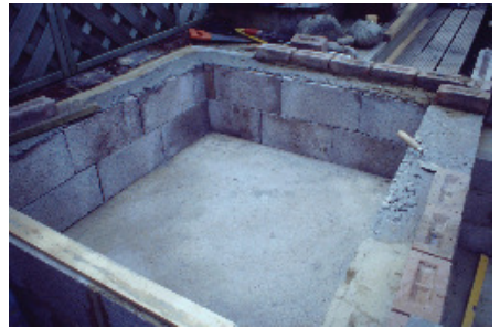
4. Building of marginal plant area
