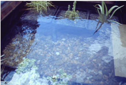
9. Liners in, planting marginal plants. 10. Filter and skimmer in place.
